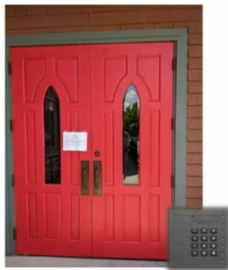
Myrtle ramp entrance
